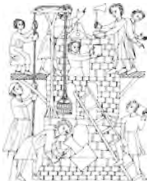
Pulley and wooden ladder (from Bible dating from the beginning of the 13th century)
