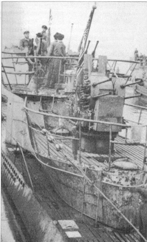
A close-up of the flak armament on U-377 after her bridge conversion. The upper platform is home to two twin 2 cm flak guns, whilst a four-barrelled Flakvierling is mounted on the lower platform. Unusually, no gun shields have been fitted to the Flakvierling in this case. (Jak P. Mallmann-Showell)
