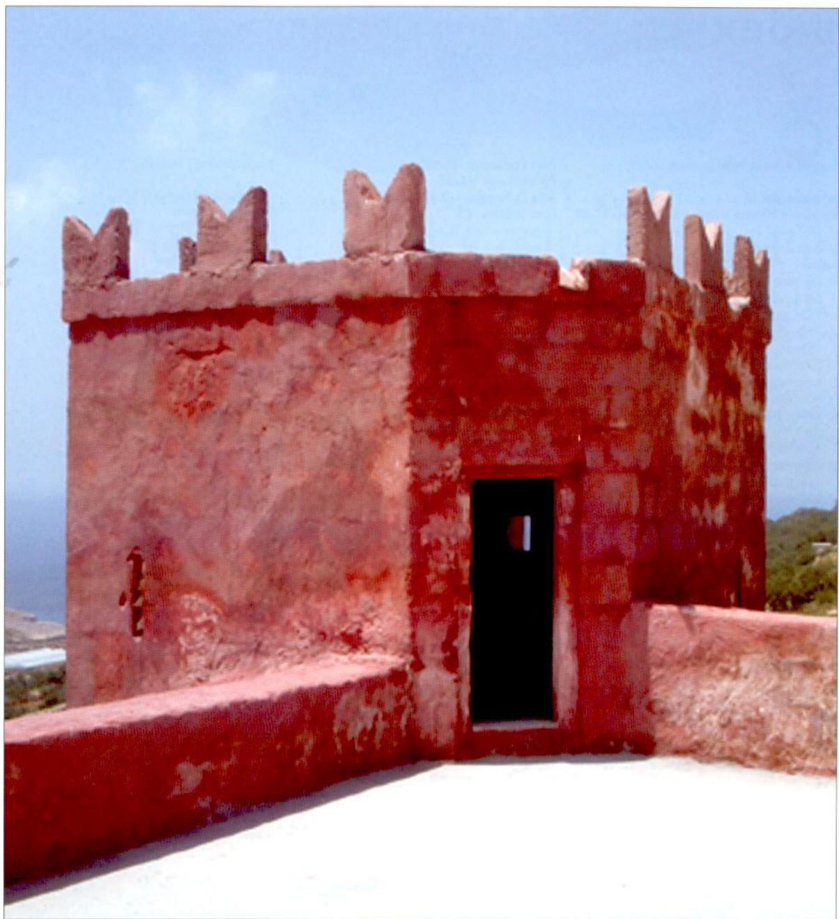
The view of the south-west turret of the Red Tower, also known as St Agatha's Tower, clearly shows the splayed merlons added to the design for decorative or, as some have argued, deterrent effect. The tower, recently restored and open to the public, is worth a visit for its magnificent views if nothing else. (Courtesy of P. Evans)
