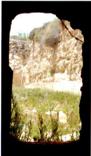
ABOVE LEFT Sunk into a drop-ditch (a ditch within the main ditch but at 90 degrees to it) this view through a caponier loophole shows the virtual impossibility of attackers being able to survive in, or get across, the main ditch. Because of the drop-ditch, the exposed portion of the caponier presented only a small target. (Courtesy of P. Evans)
