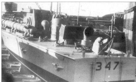
MTB 347 during the final stages of construction at the Vosper Yard in Portsmouth. One of 16 boats of this type, this 72-foot 6-inch was sunk in action against German warships off the Dutch coast in October 1944. (Vosper Thornycroft (UK) Ltd)
