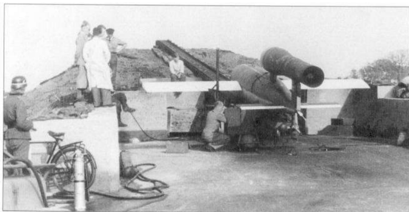
The unsuccessful Rheinmetall-Borsig launcher was replaced by a Walter design and the first prototype is seen here during trials in the autumn of 1943. (NARA)
