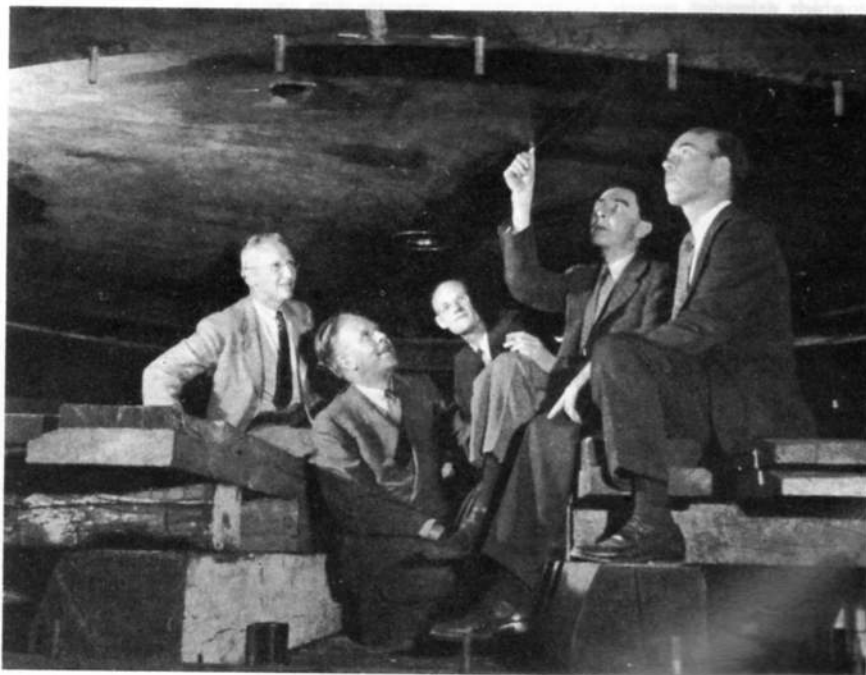
Professor Ernest O. Lawrence (second from left) beneath the pole face of the huge 4,000-ton cyclotron magnet adapted for the experimental calutron at the University of California. Scientific project director, J. Robert Oppenheimer, touches its face.
