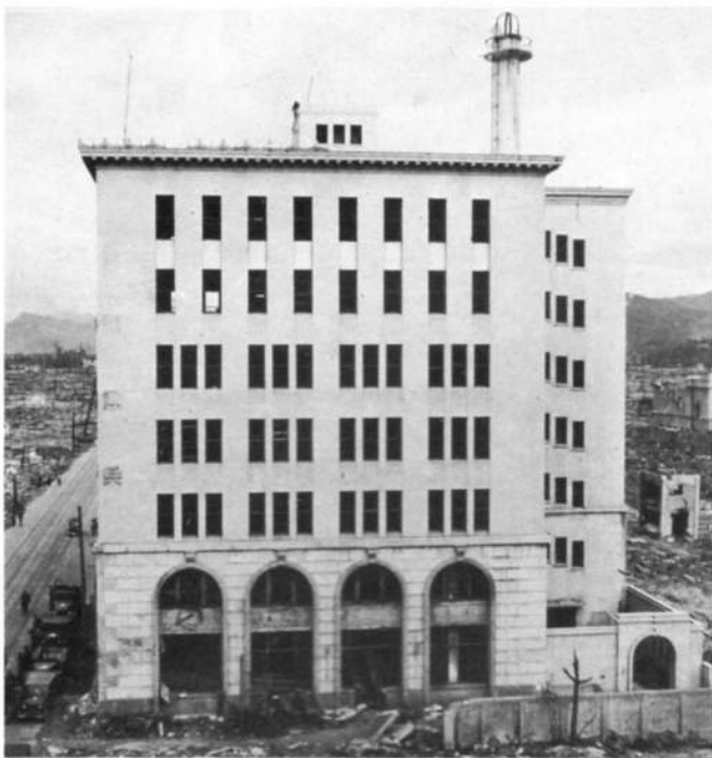
Above: The Fukuya department store, 2,500 feet from Ground Zero, was another reinforced-concrete structure which outwardly survived the blast. However direct radiated heat spontaneously ignited the interior and the fire had spread to
