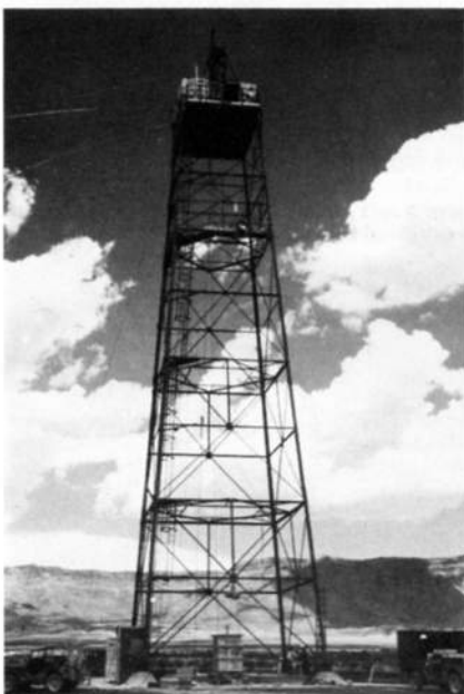
Left: It was hoped to avoid sucking up too much of the desert, which would later fall to earth as radioactive dust, by detonating the bomb at the top of a 100-foot tower.
