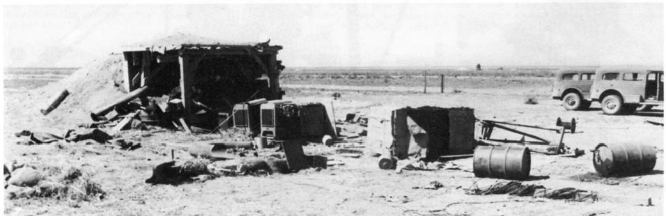
The instrument shelter damaged at North 1000 (1,000 yards from the tower). Jumbo can be seen intact in the background.
