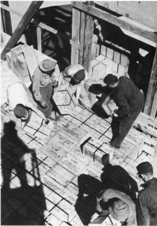
A trial run was conducted on May 7, 1945 with the explosion of 100 tons of TNT. A sturdy 20-foot tower was built about 10,000 feet south from Ground Zero and the boxes of explosive brought in from Fort Wingate. Fission products from Hanford were inserted in the stack to simulate, at a low level, the
