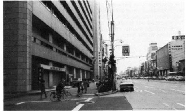
damaged, structurally roof beams were cracked and it was gutted by fire. (Kikuchi/Hirota)
