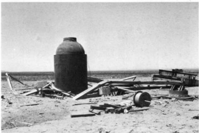
Jumbo's tower was swept away, dropping the monster without damage. After the war a series of unrelated experiments were conducted resulting in blowing the ends from the
