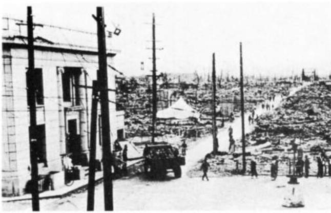
Left: The view southwards from Yokogawa Station. The bridge in the background crosses the River Tenma. (Y. Hirayama)
