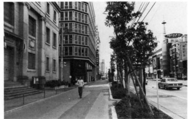
superficially damaged as the fire was restricted to one room on the south-west corner. (Kikuchi/Hirota)
