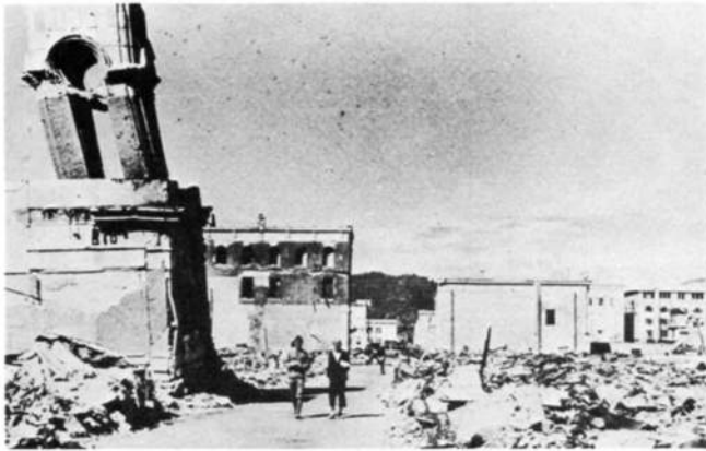
Left: The tower of the Shimomura Clock Company building leans at a drunken angle some 2,000 feet from American
