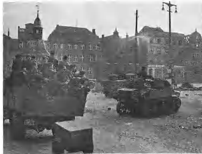
Left: The same tank wheels up the market place, while a truck-load of Luftwaffe soldiers, no doubt glad to be able to surrender to British troops, looks on. (IWM) Right: Until 1990, Wismar
