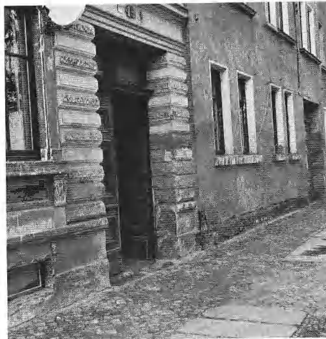
With no caption as to its location, the picture could have been taken anywhere, the most likely places being Wurzen, Trebsen, Naunhof or Torgau itself. Karel had a lucky stroke when he recognised the building as he explored Torgau. It stands on Pestalozzi-Weg (named Fürstenstrasse in 1945), the street overlooking the Elbe.
