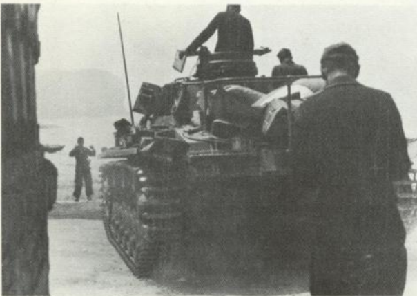
One of the few PzKpfw. III tanks of the 7th Panzer Division being guided on to a French beach at the end of the drive to St-Valéry, June 1940. Note large national flag draped over rear stowage for aerial recognition. (Conway Maritime Press)
