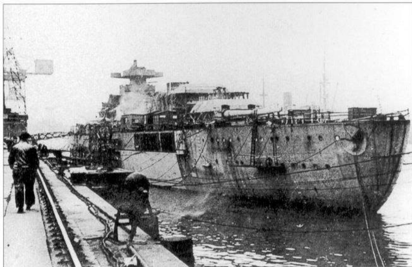
The massive turret 'Dora' can be seen in this stern view of Bismarck during her fitting out.
