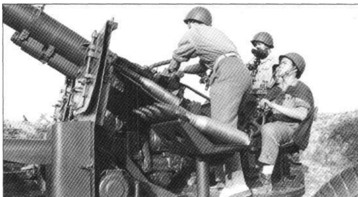
Myriad M38/39 37 mm automatic AAA guns like this one protected Kep and Yen Bai airfields. The gun's effective range was three kilometres, and it was easily transported behind a ubiquitous ZIL-151 or-157K 6x6 truck (Tran Dinh Kiem)
