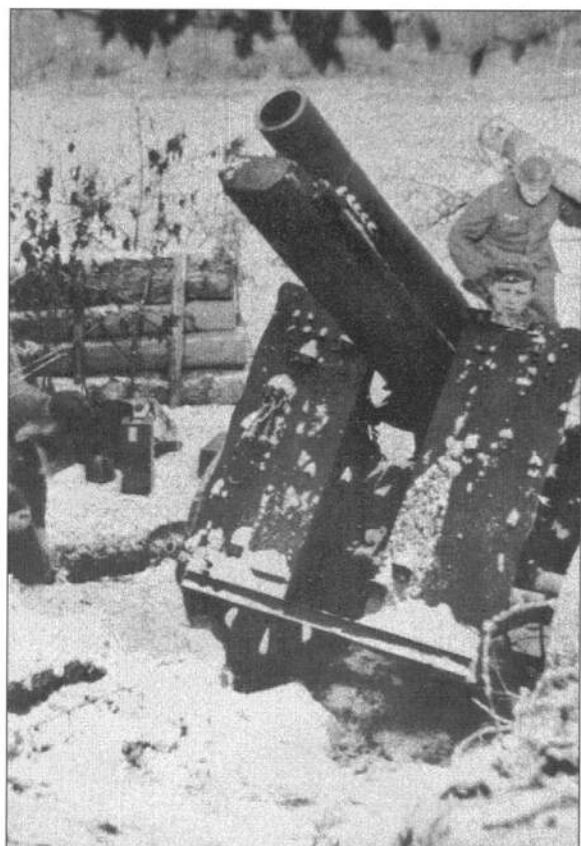
A 15cm heavy infantry gun in a log-revetted firing position. To the left of the weapon a gunner digs an armour protection trench within the position.
