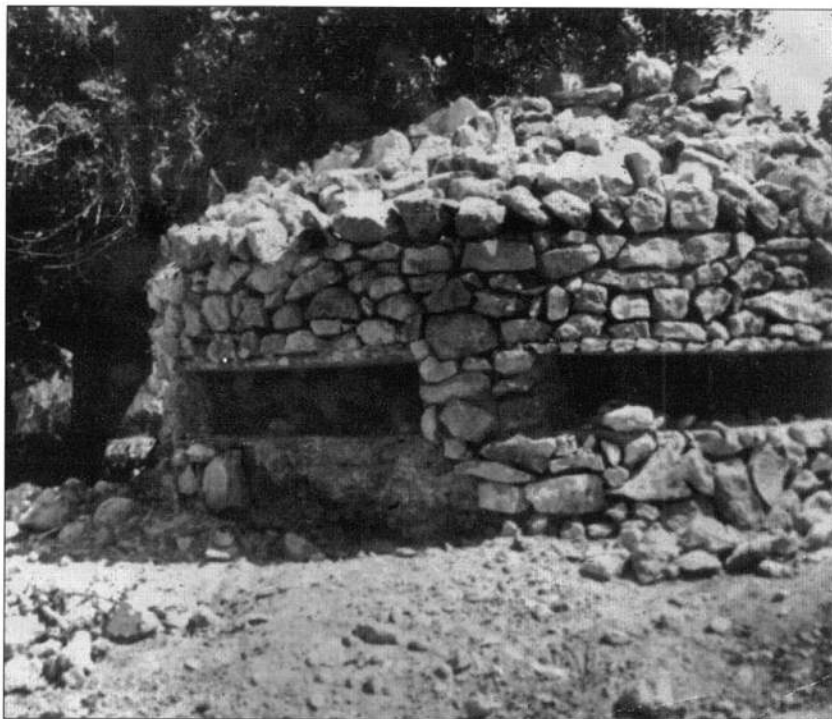
This Italian-designed, hexagonal pillbox, featuring multiple machine-gun ports, was extensively used by the Germans in Italy. Some were better camouflaged than others, blending in well with the rocky terrain. However, because the embrasures were rock-faced, machine gun fire directed into them would ricochet into the pillbox, creating rock fragments.
