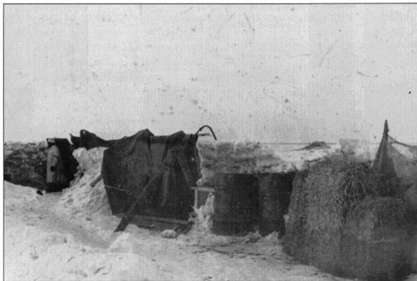
On the Russian steppes, long snow-bank barriers formed defensive lines with firing positions. Dugouts too were set in the snow berms, which were revetted with snow-filled fuel drums and hay bails (as shown here). Canvas tarps sometimes covered the dugout entrances.
