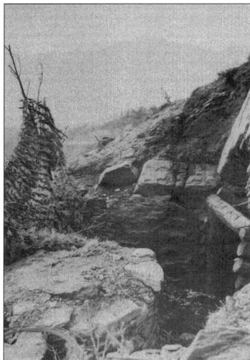
A log-reinforced dugout and rock-revetted fighting position on Mt Altuzzo, Italy, September 1944. This directed fire onto the forward slopes and across the La Rocca draw, which was an approach route. A camouflage net garnished with pine branches has been pulled away to reveal the position.
