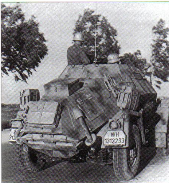
Rear details of an SdKfz 222 belonging to Panzer-Aufklärungs-Abteilung 4 in Russia, 1943. The colour scheme appears to be yellow ochre with a serpentine overspray in green. The crew seem to be wearing the green armoured car denims, and have sand-painted helmets. The 4.Panzer-Division runes, in yellow, are visible on the right rear mudguard, balanced by a white company symbol on the left. (Bundesarchiv)
