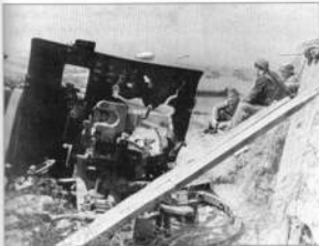
To stiffen the Normandy defenses, Rommel had pressed obsolete WWI field guns into service including German 77mm guns re-bored to 75mm and Czech Skoda 76.2mm guns. Old or not, these weapons were very effective against exposed infantry on the beaches below. This particular one has taken a direct hit, probably from a tank gun, on the right side of its splinter shield, which has also blown off one of the wheels. (NARA)
