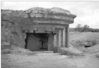
When the Rangers reached the crest of Point du Hoc, they were surprised to find that the Bauform 771 casemates were empty. The site has been preserved and this casemate was photographed by the author in the 1960s. (Author)
