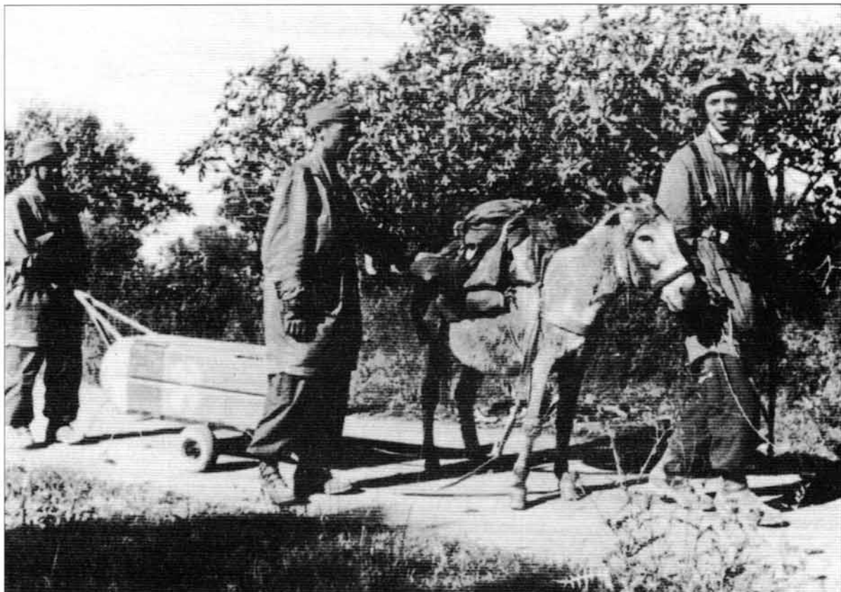
Some of the weapons containers included a small pair of wheels and a towbar, allowing them to be transformed into light handcarts, as here on Crete.
