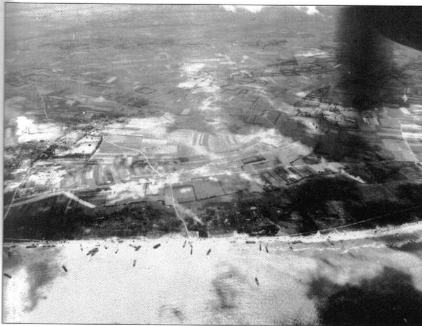
Gold Beach, King Sector mid morning 6 June. The left foreground shows the track running inland from the beach up to the Mont Fleury battery through the antitank ditch. The extreme right of the picture shows the beach curving into Jig Sector, at about the position of strongpoint WN 35 at Hable de Heurlot. (Imperial War Museum, MH 24333)
