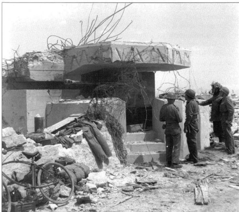
Troops from 50th Division inspect a 50mm gun in its concrete emplacement somewhere along Gold Beach. It has been struck by naval shellfire on its side, but damage seems to have been superficial. It was probably knocked out at close range by assault troops. (Imperial War Museum, B5252)
