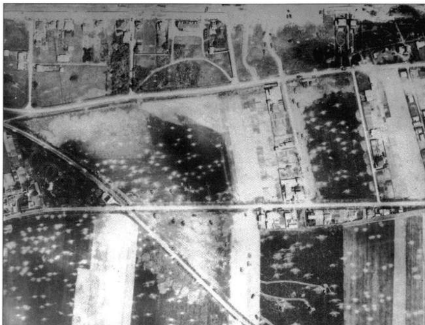
An area of Juno Beach just to the east of Bernières showing the white spotted mosaic pattern caused by the explosions of over 1,000 5in. rockets, fired by an LCT(R) out at sea. (Imperial War Museum, MH24332)
