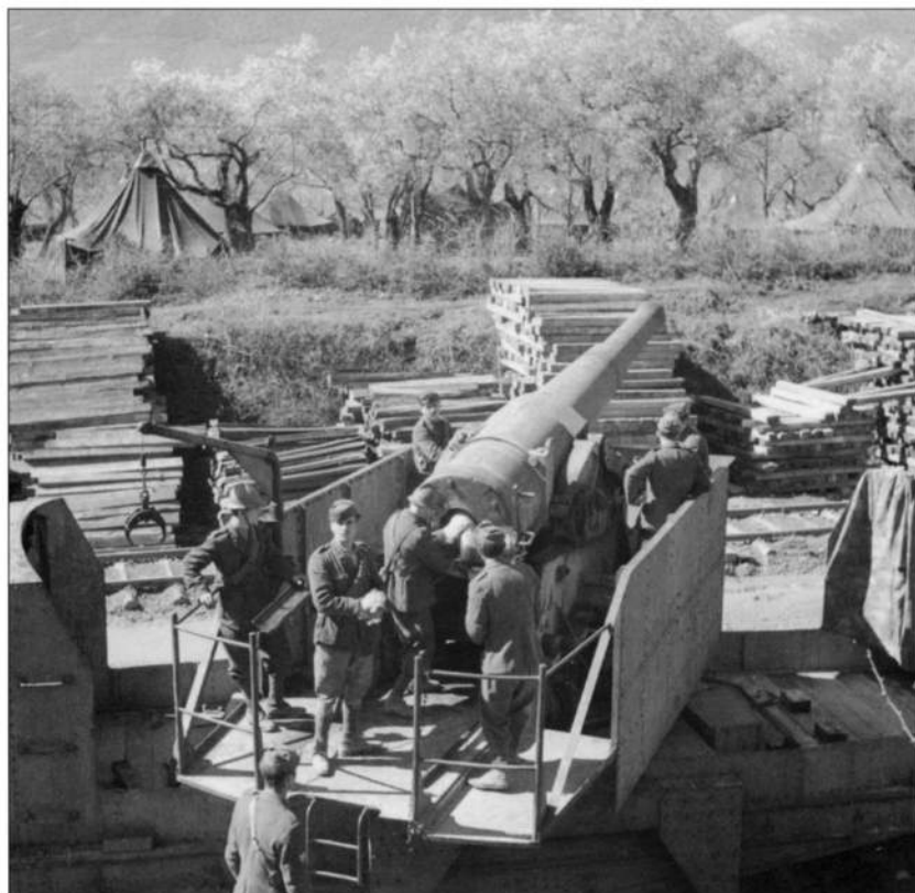
Italian 194mm railway gun of 269th Battery, Italian 1st Armoured Artillery, firing in support of Allied troops in Cassino. This battery was the only one from the regiment that had escaped the German takeover when Italy surrendered. With a range of over ten miles it was a useful addition to Allied firepower. (Imperial War Museum, NA 12848)
