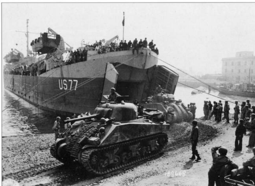
Tanks of US 1st Armoured Division are unloaded straight onto the waterfront in Anzio, soon after the main landings. (US national Archives)
