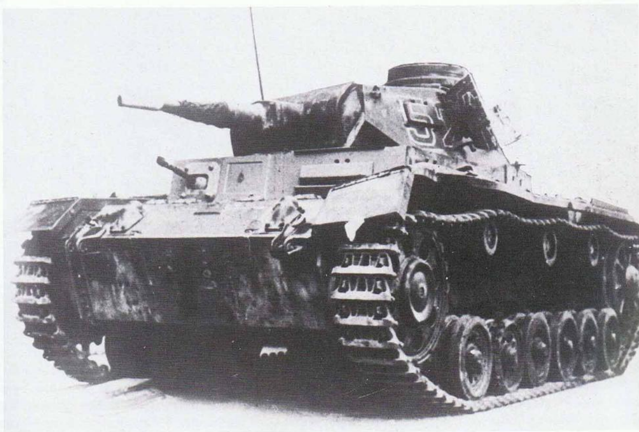
A Panzer Mark III, carrying a 37mm gun and 3 machine-guns.
