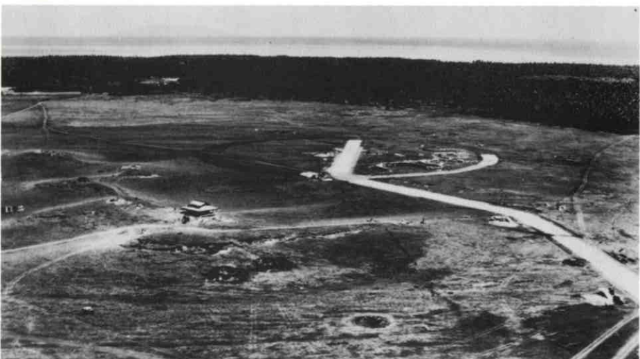
◀ Taxi-way to main runway is clearly defined, as are circular plane revetments. The structure to left is the pagoda type control tower that was set up by the Japanese to control airfield operations. The preparations made on the ground are clearly indicative of how far the Japanese had progressed to complete the airfield. (USMC)
