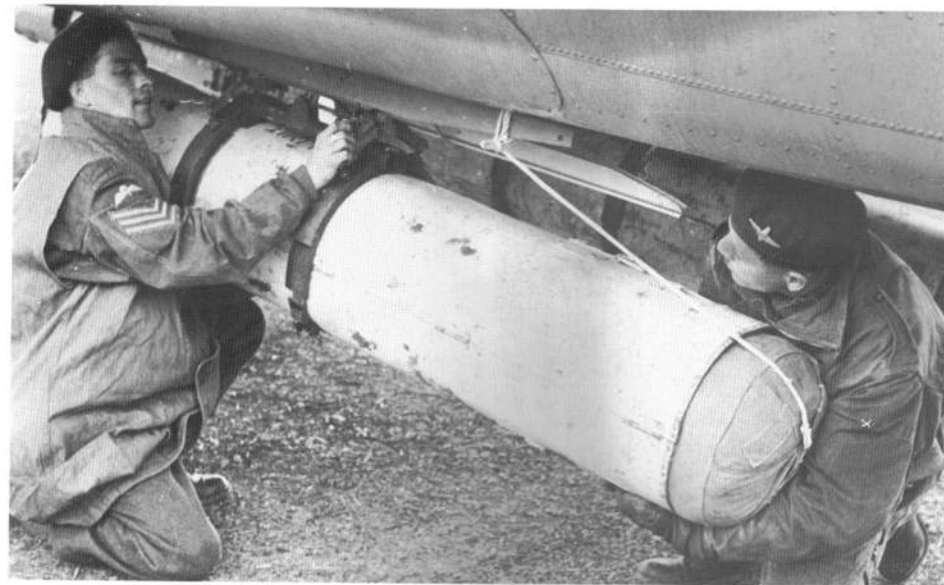
▲ Two British paratroops, one of them wearing the sleeveless 'jump jacket', fit a Mark I Weapons Container underneath an aircraft before take-off in England. Fitted with its own parachute, this
