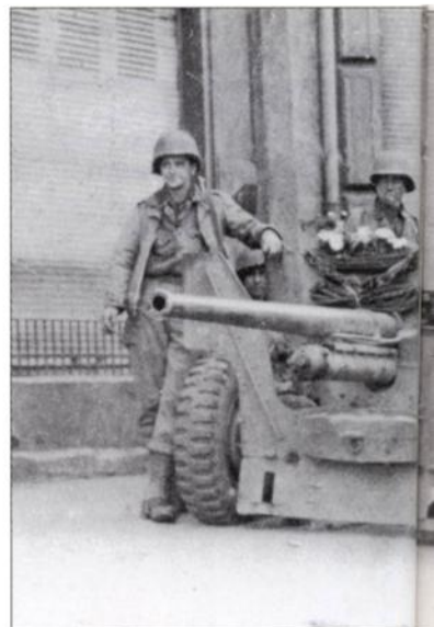
ABOVE An M1 57mm anti-tank gun covers an intersection in Algrange during the fighting between the 358th Infantry of the 90th Division and the 559th Volksgrenadier Division on 10-12 September. The 57mm gun was a license copy of the British 6-pdr anti-tank gun and was the standard anti-tank weapon of infantry divisions in 1944. There were 18 in each regiment, three per battalion. The 90th Division also had an attached towed
