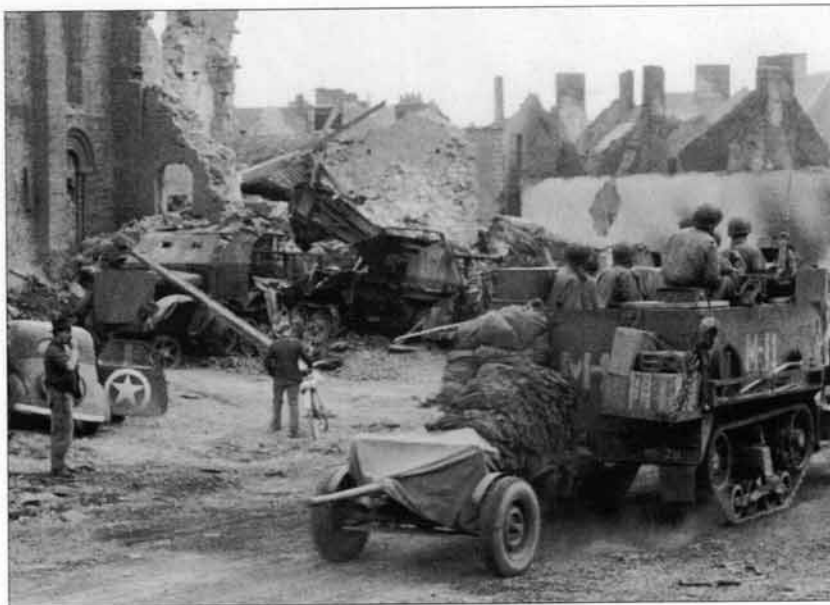
LEFT An M3A1 half-track of the 2nd Armored Division passes by some of the wreckage in Roncey on 1 August. This is a view from the other end of the church and an armored SdKfz 7 half-track fitted with a quadruple 2cm anti-aircraft cannon can be seen near the wreck of a Marder III of the 17th SS Panzer Grenadier Division.
