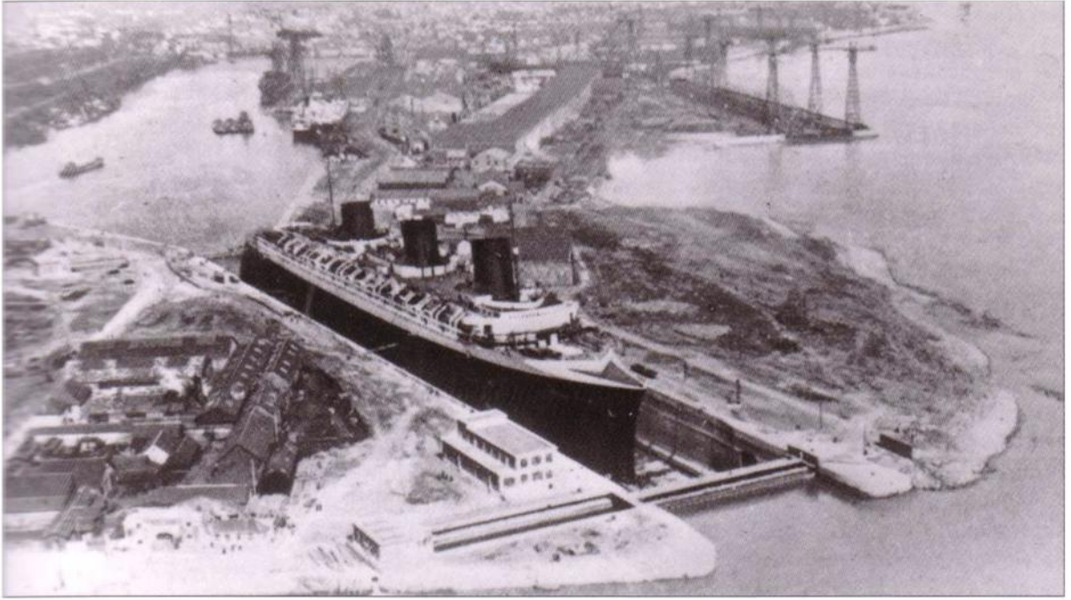
The liner Normandie , the pride of the French maritime fleet, in the massive dry dock in St Nazaire before the war. In the foreground is the winding shed with the long water-filled camber linking it to the outer caisson of the dock. The dock was opened by pulling the caisson on its rollers back into the camber. Immediately behind the camber is the pumping house. The dry dock also served as a lock, linking the Penhoët Basin with the River Loire. (Imperial War Museum, HL 53265)
