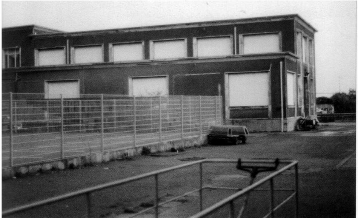
The pumping house alongside the Normandie Dock, the target of Lt Chant and his demolition team. (Author)
