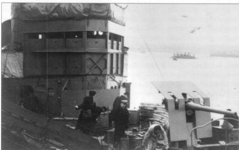
LEFT, CENTRE Steel plating has been welded to Campbeltown's wheelhouse to give some protection from smaller calibre weapons. The forward 4in. gun has been replaced by a quicker-firing 12-pdr. (Imperial War Museum, HU53259)
