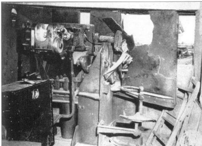
This 50mm anti-tank gun in the Bauform 667 casemate was knocked out by a direct hit on its shield by tank gun fire. These ferro-concrete bunkers were nearly impervious to bombing and naval gunfire, and had to be eliminated by close combat assault. (USAOM)
