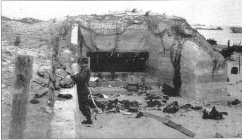
One of the most effective types of bunker on the Normandy coast was the Bauform 667 casemate, which were positioned parallel to the shore to permit enfilade fire along the beach. This Bauform 667 casemate of the W5 strongpoint at Utah Beach was armed with a 50mm anti-tank gun, and it was knocked out by tank gun fire directed against the embrasure from close range. (NARA)
