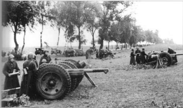
The mechanisation of two Polish cavalry brigades led to some modernisation of the field artillery. The standard French Mle. 97 75mm gun was made suitable for motorised traction by the addition of a new suspension and pneumatic tyres. This particular battery served with the 10th Mechanised Brigade. (J. Magnuski)
