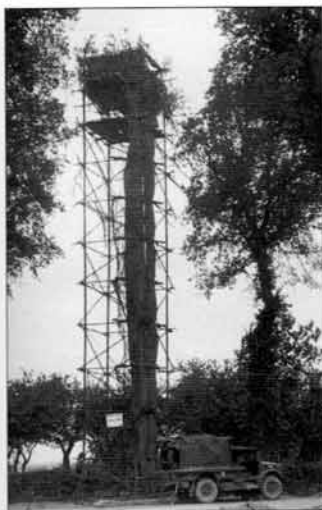
This 66ft-high observation tower was erected on high ground north of Cheux by VIII Corps Royal Engineers for 10th Survey Regiment Royal Artillery. Its observers were attempting to spot the flash of enemy guns near Verson and Hill 112 so that they could be targeted with counter-battery fire. (IWM B7043)
