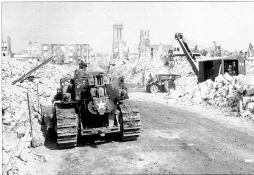
Royal Canadian Engineers clearing rubble from the streets of Caen. It was important to get roads opened quickly so that troops and tanks could get forward to the bridges over the Orne in the city. (Ken Bell, NAC 169342)
