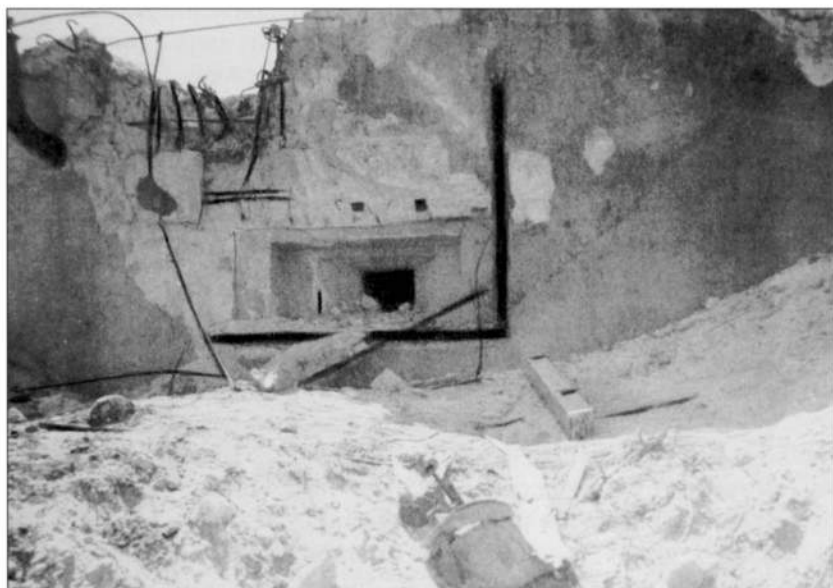
On each corner of Roi Island were 40ft-diameter (12.2m) concrete blockhouses mounting 7.7mm Type 92 heavy machine-guns. This one had sustained several direct hits by large-caliber naval guns, but survived until knocked out by Marine assault teams.
