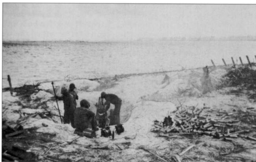
75mm M1A1 pack howitzers of the regimental cannon companies were landed in later waves and set up to fire across the lagoon at the north curve of Kwajalein.
