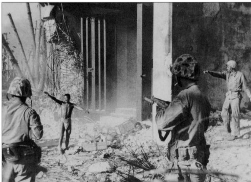
Marines flush prisoners from a concrete blockhouse. The tangle of torn reinforcing bars indicates a direct hit, but the massive steel doors remain intact.
