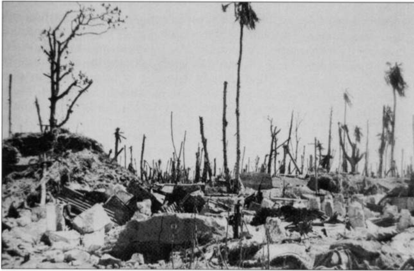
Many of the scores of concrete structures on Kwajalein were completely destroyed during the repeated pre-invasion bombardments. The numerous structures on "Burton" (Ebeye) Island to the north of Kwajalein suffered a similar fate.
