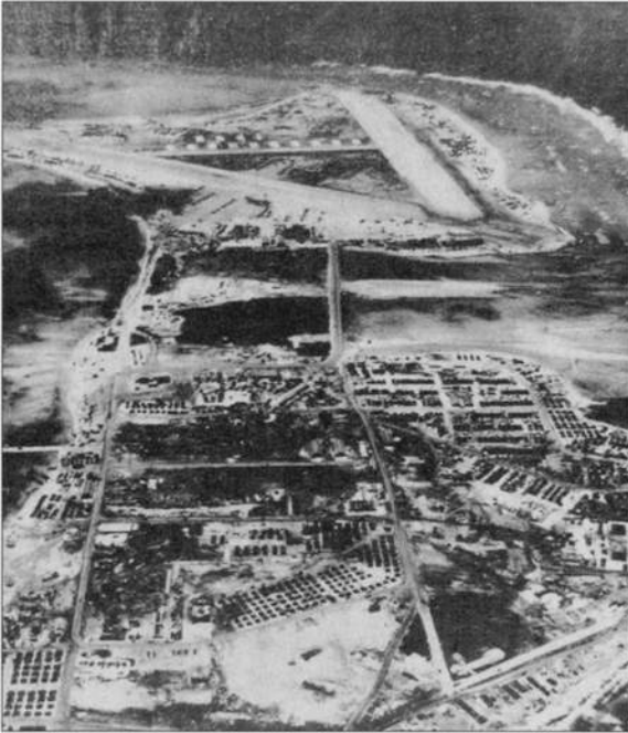
ABOVE Roi-Namur after being completely rebuilt by Seabees and established as an airbase. As with many such conquered islands, it was virtually stripped and leveled as extensive base facilities were constructed.
