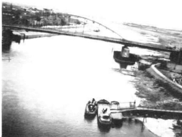
Rare aerial reconnaissance photo of the Arnhem road bridge, taken on 6 September 1944. Note the open ground to the south of the river (right); and the built-up area to the north (left), in which 2 Para made their heroic stand two weeks later. The bridge was destroyed by the Germans shortly before they withdrew from Holland in 1945. (ABF Museum)
