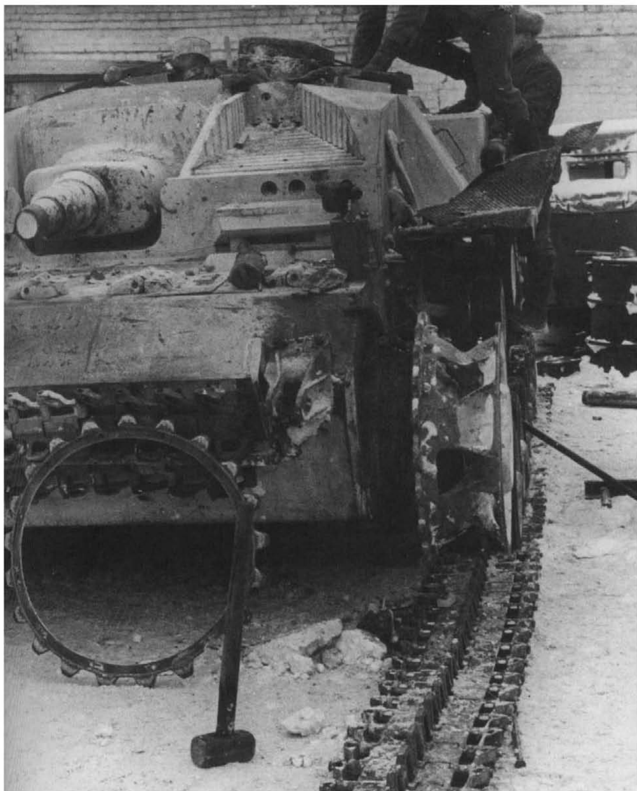
A Sturmgeschütz Ausf. B at a repair depot after retrofitting the Sfl.ZF1 sight that was originally introduced at the
