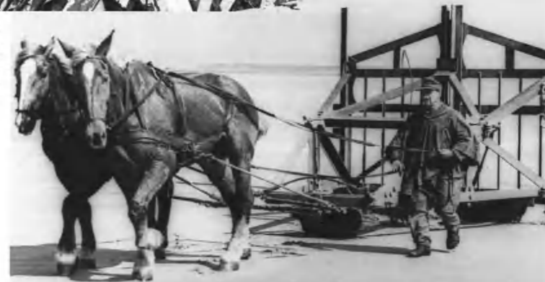
Right: A 'Belgian Gate' (also known as 'Element C'), being dragged along the beach at low tide. These mobile obstacles were some 3m high and 3m wide. Bundesarchiv
