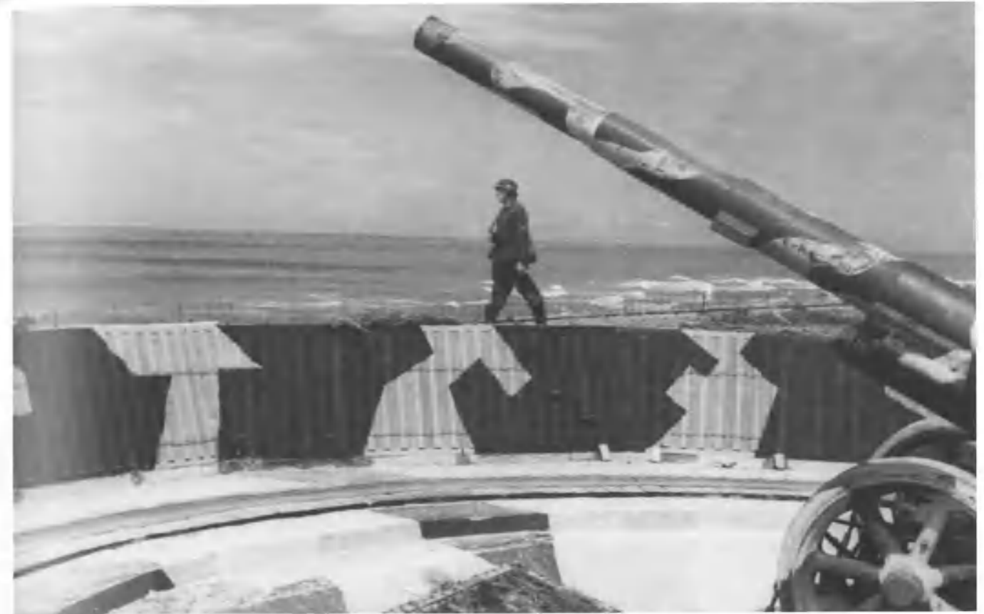
Above: Somewhere on the Belgian coast was this camouflaged gun position containing a Feldkanone 418(f). Note the all-round traverse, which had to be set by hand, three of the gun crew pushing the heavy 10,000+kg gun around — not an easy task. Bundesarchiv
