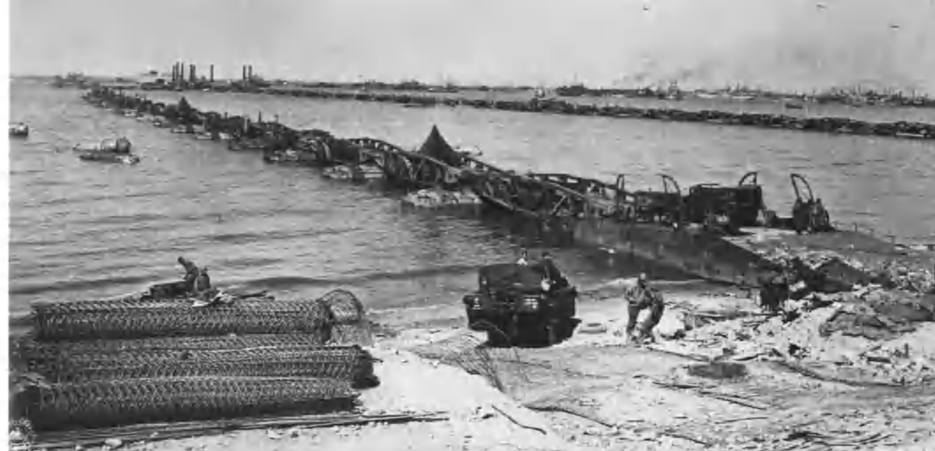
Above: This was one of the two 'aces up the Allied sleeve', namely the pair of prefabricated Mulberry Harbours, which were towed over to the Normandy beaches, thus reducing the need to capture an intact port. This photograph was taken before the severe gales that wrecked one of the two harbours. US Army
