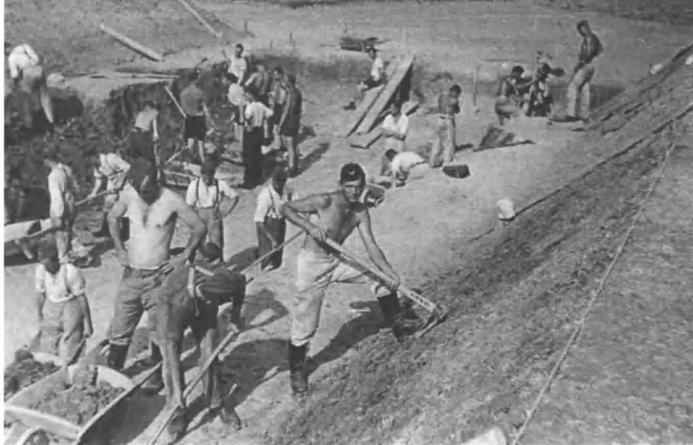
Above: Divisional field engineers had a wide range of duties, including the construction of obstacles, whilst Army construction battalions were responsible for reinforced field-type constructions. These soldiers are hard at work building defences on the coast of Normandy in 1943. J. P. Benamou Collection
