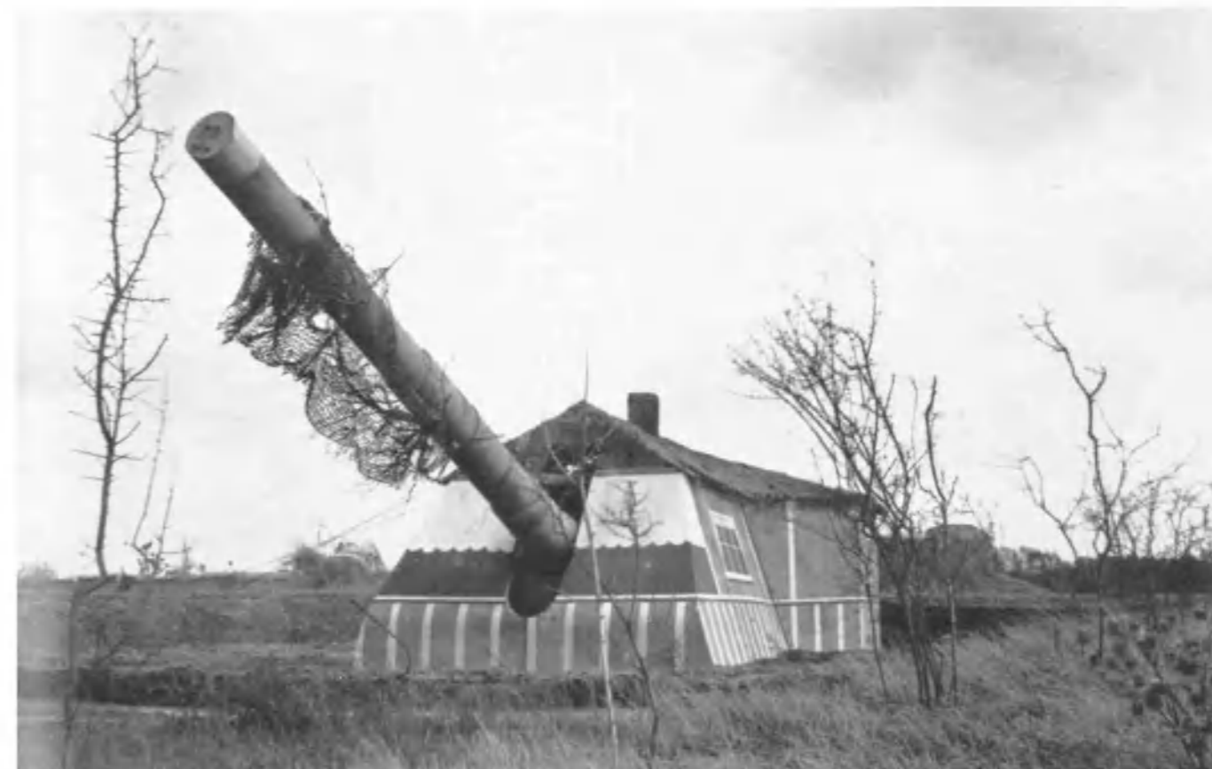
Above: Is it a house or is it a gun emplacement? Largest of the guns on the Channel Islands were those of the Mirus Battery, which comprised four reconditioned 30.5cm guns off a World War 1 Russian battleship. These were located at St Saviour's, Guernsey. IWM — HU 29057
