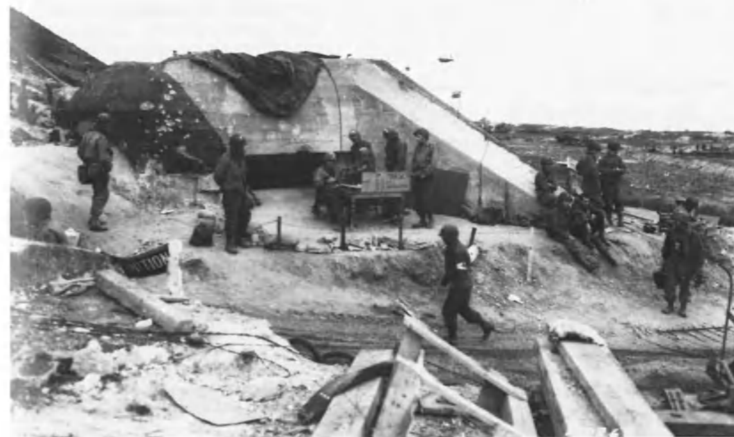
Left: This captured enemy blockhouse which protected the E-1 draw (west side) has become a temporary HQ for the Engineer Special Brigade Group. This unit operated Omaha Beach as a port of supply until December 1944. Postwar, the blockhouse became a battle monument. US Army via Real War Photos
