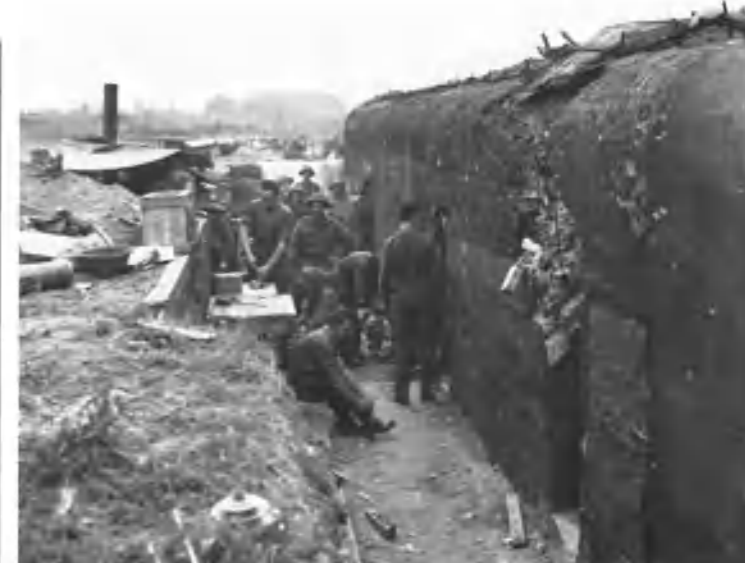
Above: A slightly damaged Type 622 accommodation bunker at Carpiquet now housing Canadian troops. Ken Bell, National Archives of Canada PA141708
