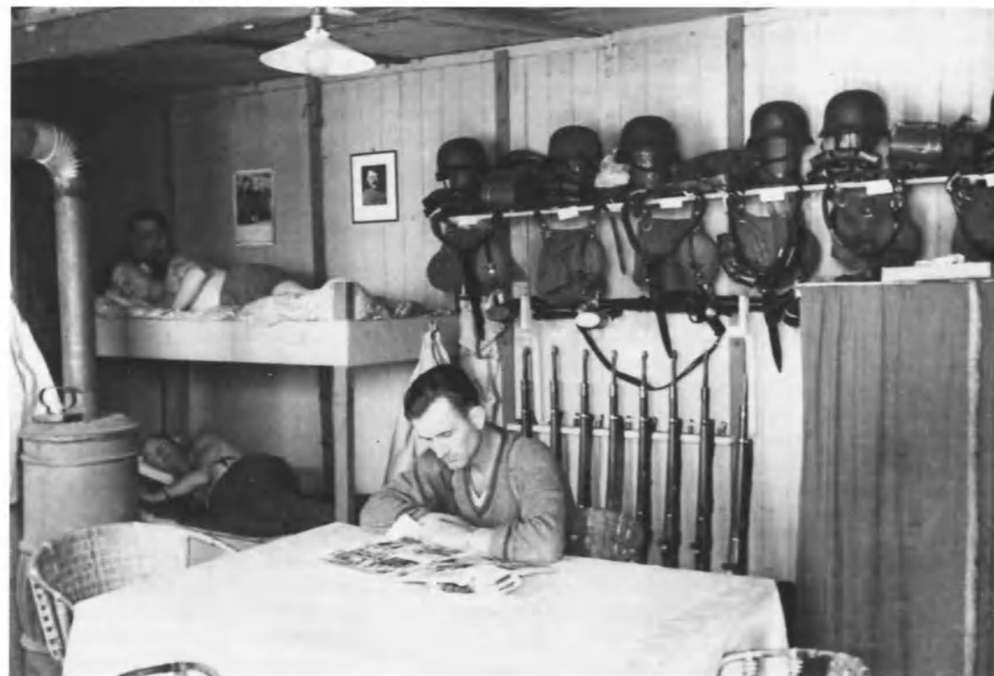
Right: Inside one of the infantry Gruppe bunkers, designed to hold a squad/section of 10 men. Note the racks for their rifles, steel helmets and personal equipment, the two-tier bunks and the coal/wood-burning stove, also the electric light. Their only 'pin-up' appears to be Adolf Hitler! The bunker was at Zeebrugge. Bundesarchiv
