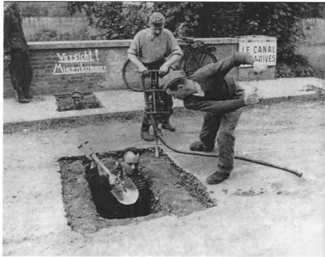
Right: Army engineers mining a bridge over the canal at Troarn, south-east of Caen. J. P. Benamou Collection
