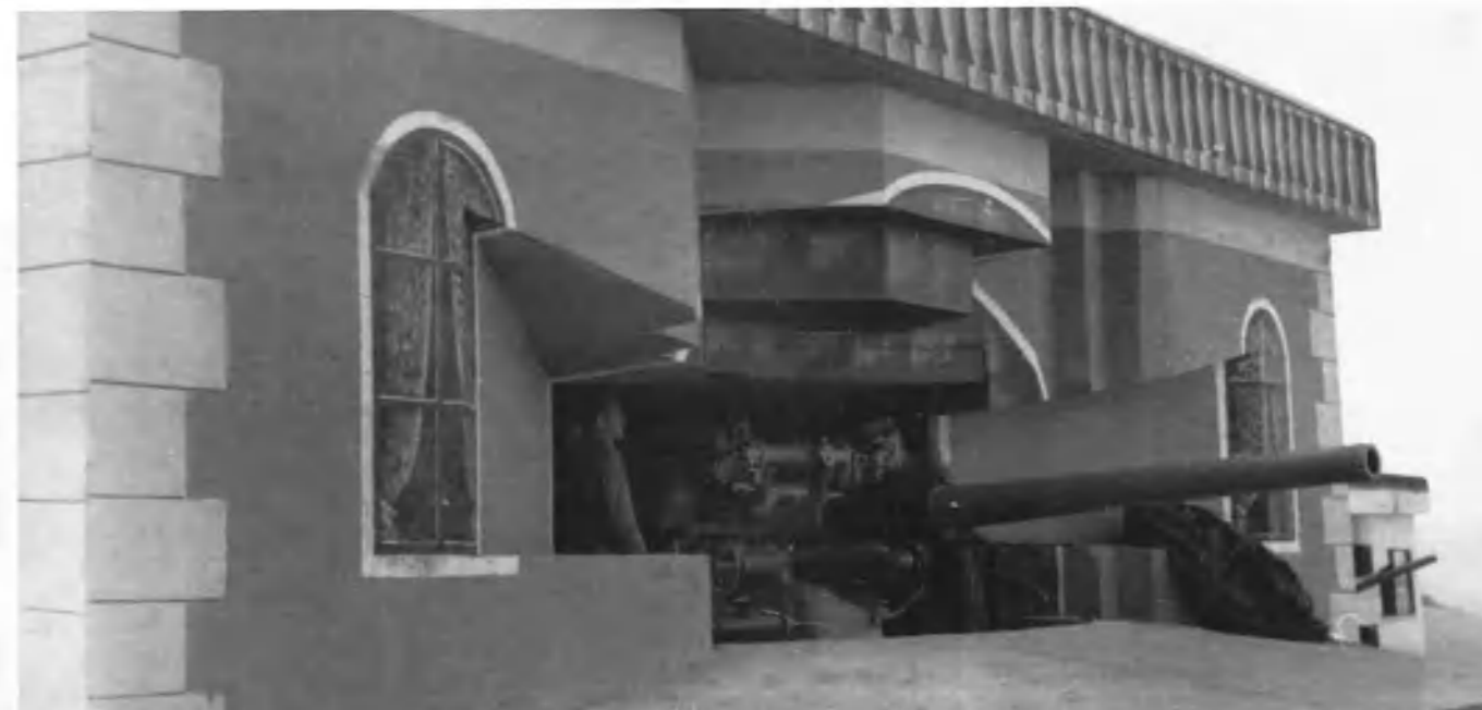
Above: This German gun position has been camouflaged to look like a seaside villa, complete with painted windows and curtains. Bundesarchiv
