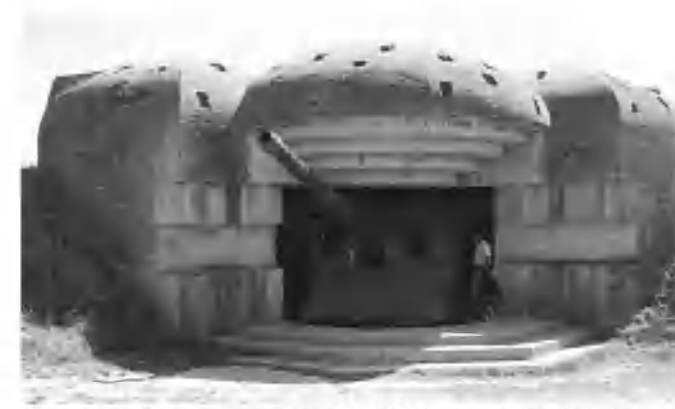
Above: One of the four gun positions (Type M272 bunkers) belonging to the Longues-sur-Mer battery still has its 15cm C/36 torpedo boat cannon in position. There was also a 122mm K/390/1(r) gun for illumination. Jonathan Forty
