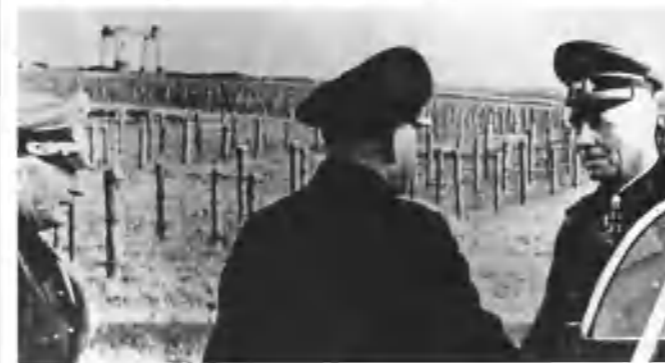
Above: Rommel and his 'asparagus' — anti-paratroop and anti-glider-assault stakes, which he had caused to be erected in as many open, vulnerable places as possible. IWM — HU3066
