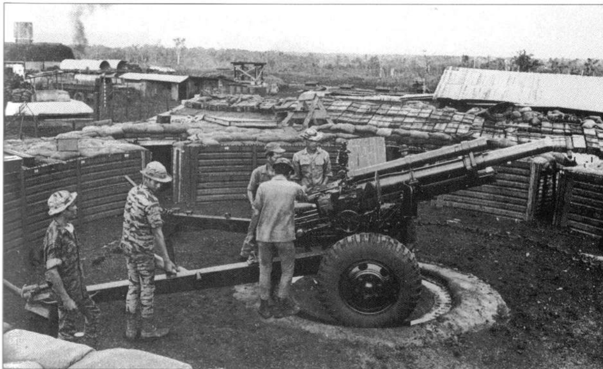
The background of this well-built CIDG-manned 105mm howitzer position provides an excellent example of the general appearance of a typical CIDG camp, here Camp Bu Dop, A-341. Camps were a mix of new construction and rundown structures, some of crude appearance. The gun position's sides are revetted by olive-drab steel airfield planking. The World War-Two-style pierced landing matting was also used.
