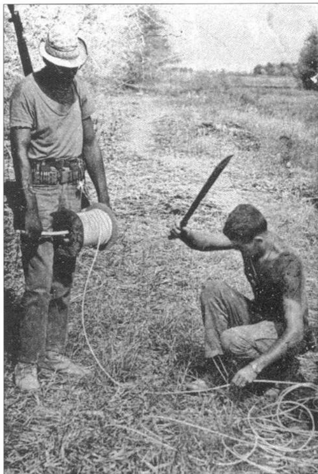
Two SF engineer NCOs cut a length of detonating cord to prepare demolition materials in order to clear trees hampering the approach to Camp Duc Hue's A-325 airfield. One man carries an M1 rifle with an M2 flash hider.
