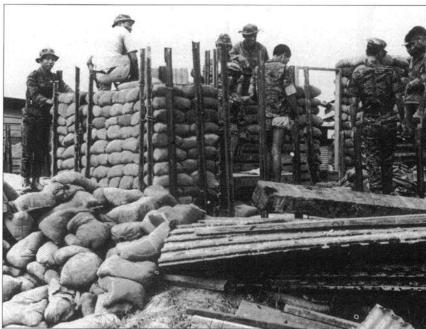
SF NCO and Strikers replace a bunker destroyed in an attack, Camp Dac Hue, A-325. Distorted airfield landing planks and timbers from the destroyed bunker are in the foreground. Some of those materials will be reused in the new bunker. Olive-drab U-shaped barbed wire pickets brace the new sandbag walls.
