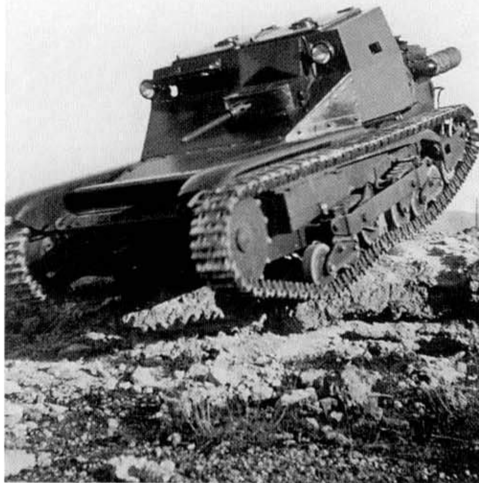
A Carro Veloce 33 pilot vehicle rolls down a rocky hill during its 1933 acceptance trials. This tank fell more properly within the tankette classification, with a weight of 3.4 MT (3.8 tons). Early CV 33s (later designated L 3-33s) were armed with one 6.5MM Fiat-Revelli Model 14 air-cooled aircraft machine gun.
