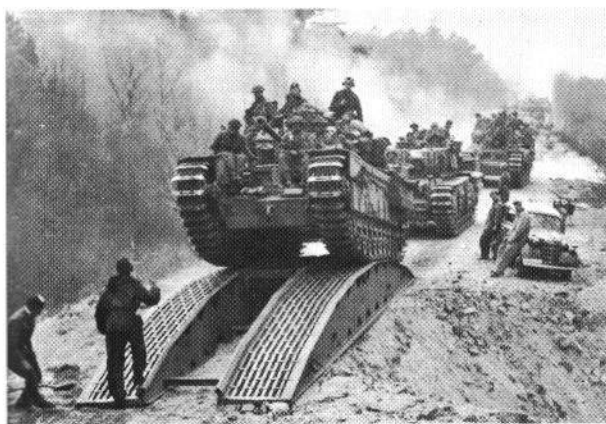
The 30-foot bridge carried by the Churchill bridgelayer was also used to reinforce cratered roads.
