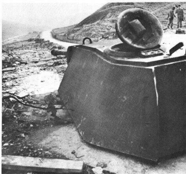
Carefully sited Panther turrets on concrete casemates were encountered in the Hitler and Gothic Lines.
