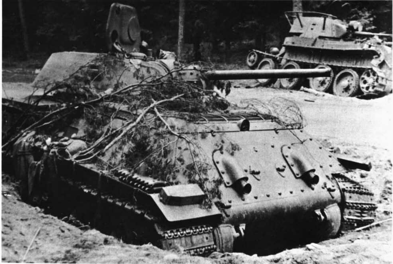
The early mechanized corps which fought in the Brody-Dubno battles were equipped with a mixture of vehicles like this T-34 Model 1941 with the new long-barrelled F-34 gun, entrenched in the foreground, and the older BT-8TU in the background. (Charles Kliment)
