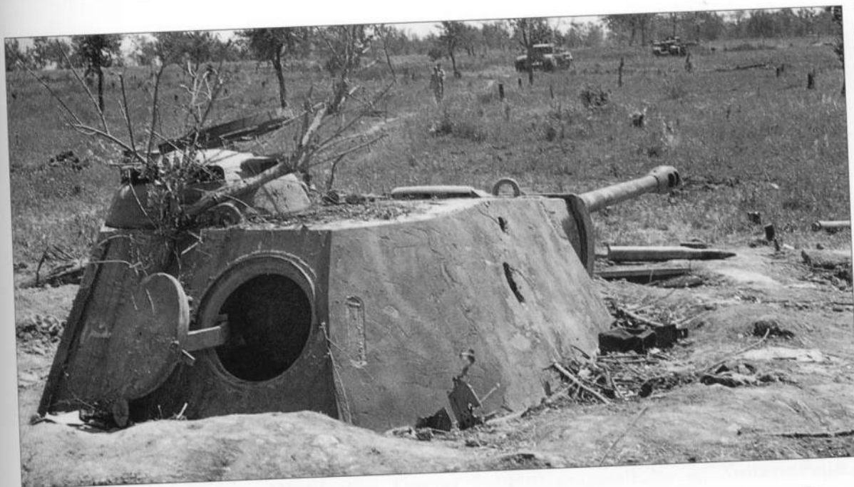
This Panther Ostwallturm was part of the Hitler line in Italy and was positioned near Monte Cassino. It consists of a normal Panther turret mounted on the Stahluntersatz (steel sub-base). Some of the Churchill tanks which it destroyed can be seen in the distance. (Imperial War Museum)
