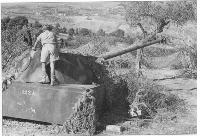
This Panther Ostwallturm was abandoned before it could be mounted on its crew quarters sub-base. It was to be part of the Gothic line in Italy and was photographed in September 1944. The turret was specially produced for static deployment, with 40 mm roof armour and a hatch with a rotating periscope instead of a cupola. (Imperial War Museum)
