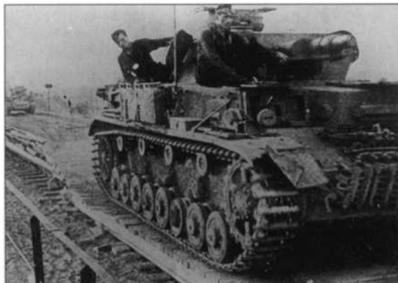
Russia 1941. A PzKpfw IV of an unidentified unit crosses a railway bridge, using additional decking laid by engineers to protect the track beneath.
