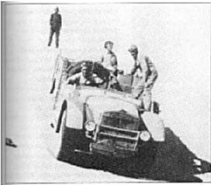
'Shooting a dune' during training with a captured Italian Fiat SpA AS37, apparently in its original scheme of grey stripes. Twelve of these trucks, booty from Operation 'Compass', were used upon formation by first S, and later Y Patrol. Although originally issued to enemy Auto-Saharan companies, they proved mechanically unsound when the LRDG put them through their paces with three weeks' stores on board. Training crews seem to have adopted overalls and MT goggles throughout - perhaps because they were continually having to 'get out and get under'!
