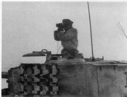
Photographs of the Panzerbefehlswagen Tiger are rare. This photograph shows a Panzerbefehlswagen Tiger built in January February 1944. It has no M.P. Stopfen in the turret side, but the Nahverteiligungswaffe (Close in defence weapon) has not yet been fitted. The 2 meter rod antenna on the turret roof is for the FuG 5 transmitter/receiver mounted in place of the
