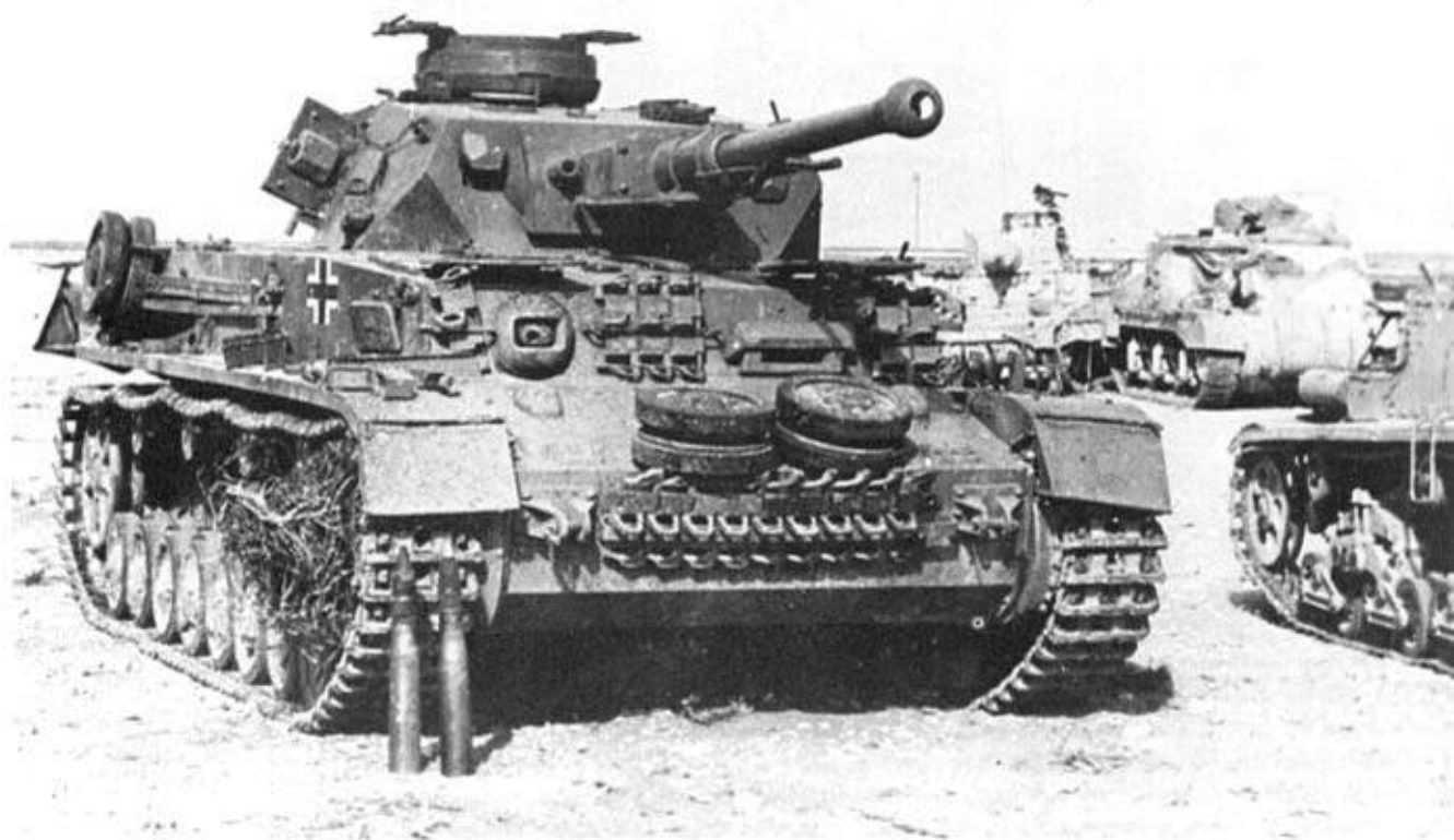
Above: In company with Allied Honeyys and Grants in this Desert tank park is a captured PzKpfw IV Ausf F 2, the first type of PzKpfw IV to mount the long-barrelled 75mm gun. Note the early single-baffle muzzle brake. (TM)
