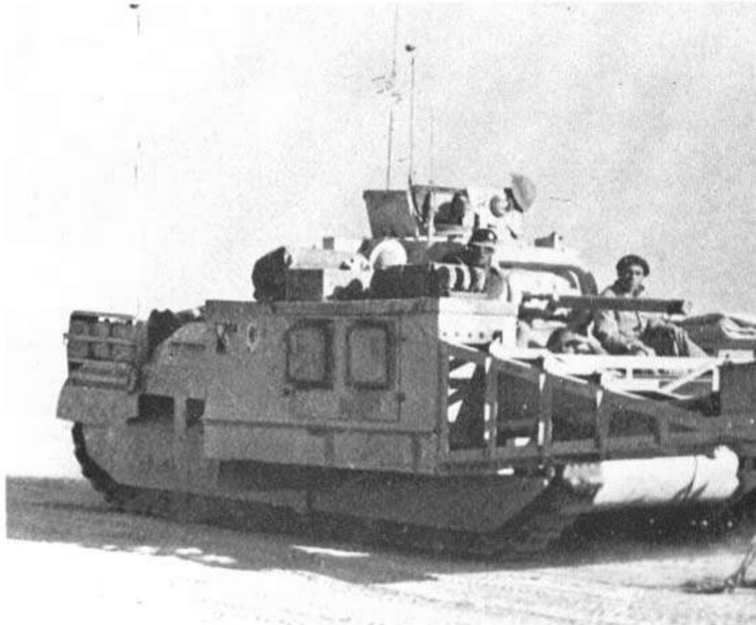
Right: Matilda II equipped with an early Scorpion Mk I mine flail, designed and produced between 1942 and 1943. The drum was driven by a auxiliary engine with the operator seated alongside. The Scorpion Mk II, had better side beams and was operated from inside the tank. (TMO)
