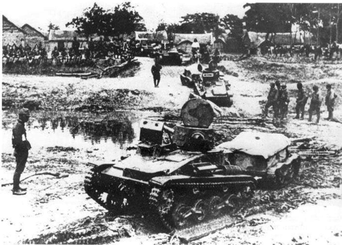
Above: These tankettes, fording a stream in China, are towing light tracked trailers. A diesel version of the Type-94 TK was built but only as a prototype. (TAM)
