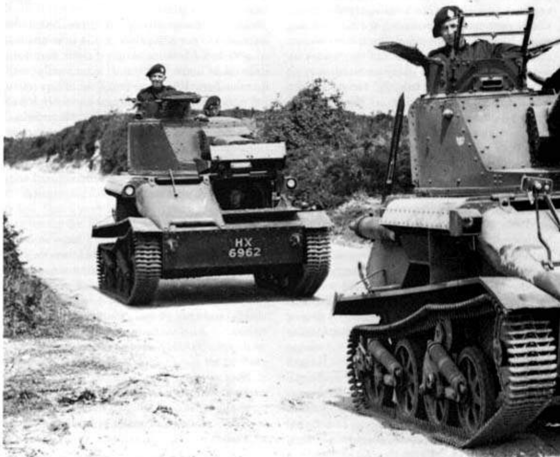
Above: A Light Mk IIB (India pattern) on trials in India, 1935. These little tanks did extremely well, especially over the rough terrain of the North West Frontier. Note the square-shaped non-rotating cupola on top of the turret. (TM)
