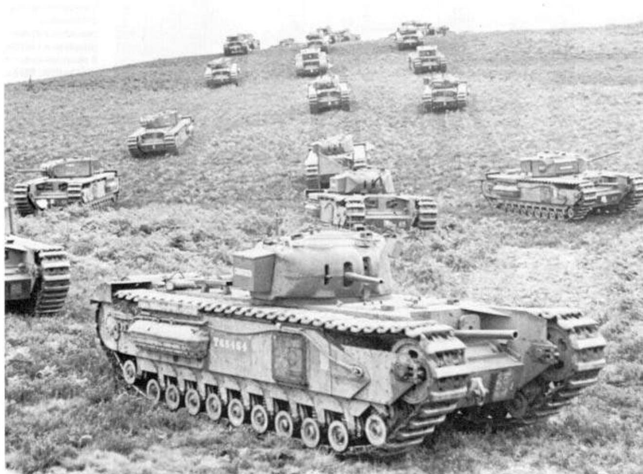
Above: Early Churchills on a training exercise in the New Forest, England - leading is a Mk I with a nose mounted 3-inch howitzer, others are Mk IIs with the howitzer removed and replaced by a BESA machine gun. (TM)
