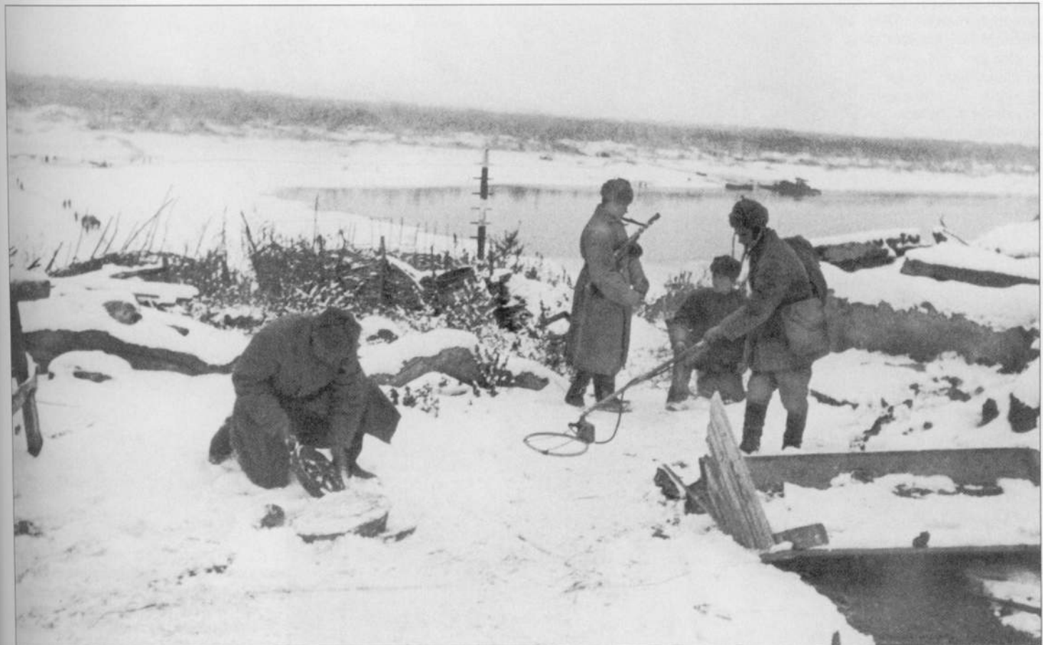
This photograph, which was taken outside the village near a lake, shows more sappers removing mines from a road.
