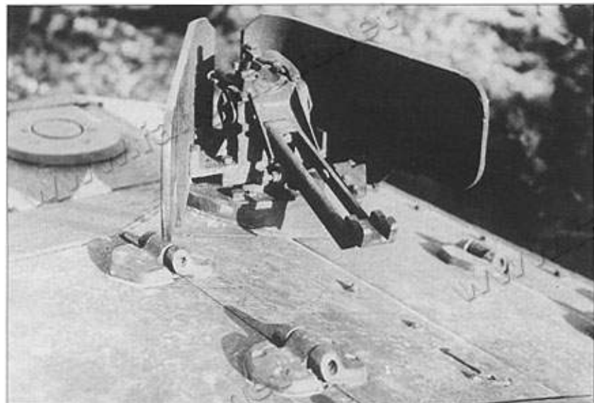
Close-up detail of the Rundumsfeuer (remote controlled) machine gun mount introduced in April 1944. Forward of this mount is the Nahverteidigungswaffe close-defence weapon that was fitted in some Sturmgeschütz from May 1944 and in all from October 1944. (HLD)
