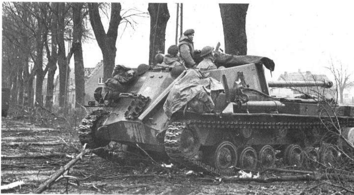
Above: The highly effective Valentine Archer SP gun, mounted a 17 pounder gun, and was one of the best anti-tank guns of World War Two. Here one guards a road near Nutterden, south east of Nijmegen, Holland during the Rhine offensive, in early 1945. (TM)
