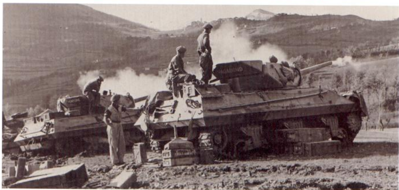
Below: M10s were sometimes used to provide artillery support, especially when there were shortages of conventional artillery. The 3-inch gun had a maximum range in excess of 14,500metres and fifty-four rounds were carried on the vehicle. (TM)
