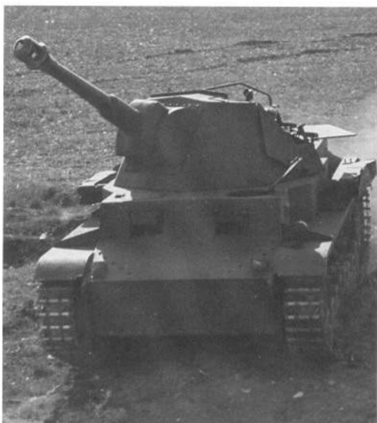
Above: The 10.5cm leFH18/1 L/28 auf Waffenträger GW IVb, was better known as the Heuschrecke (Grasshopper) 10. Only three prototypes of this tracked light field howitzer were built in 1943. (TM)
