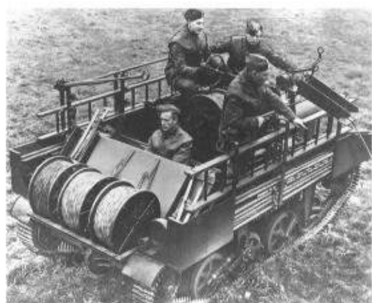
Right: Carrier Tracked Mechanical Mk1 fitted with three drums of cable and cable feeder. (TM)
