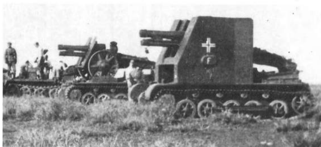
Above: The 10.5cm leFH18/1 L/28 auf Waffenträger GW IVb, was better known as the Heuschrecke (Grasshopper) 10. Only three prototypes of this tracked light howitzer were built in 1943. (TM)
