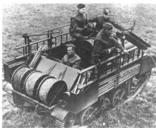
Right: Carrier Tracked Mechanical Mk1 fitted with three drums of cable and cable feeder. (TM)
