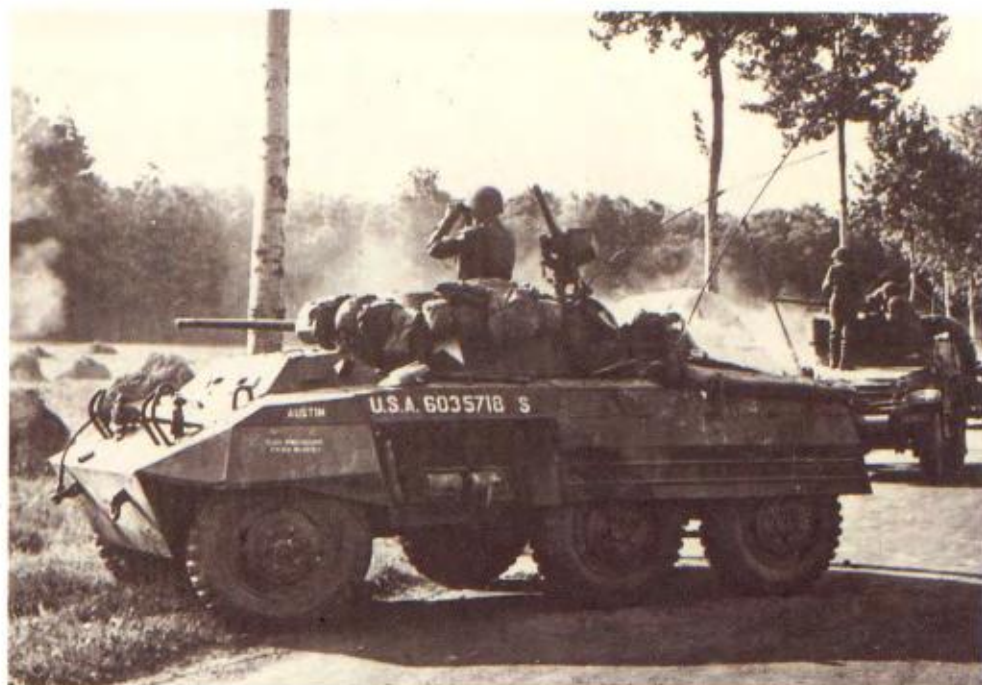
Below: The M8 Greyhound was the only armoured car to be used by the US Army in large numbers. Over 8,500 were built by the Ford Motor Company.
