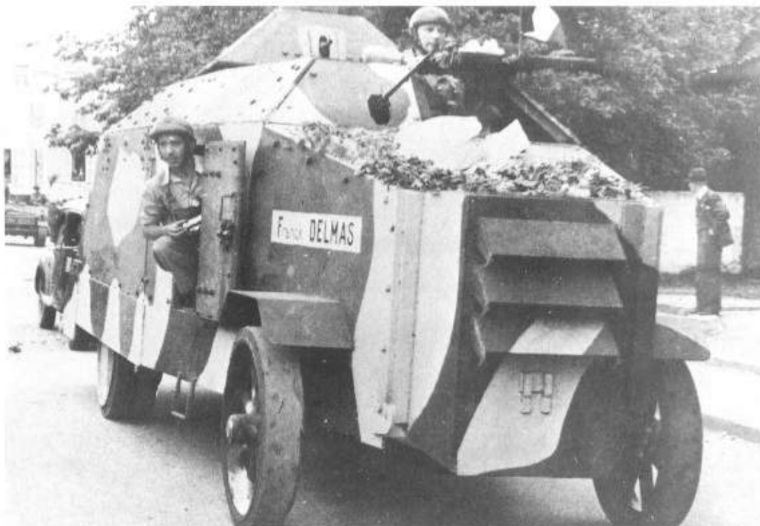
Right: An improvised armoured car used by French Resistance fighters against the retreating Germans. The solid rubber tyres show that it was built on an early lorry chassis. (TM)
