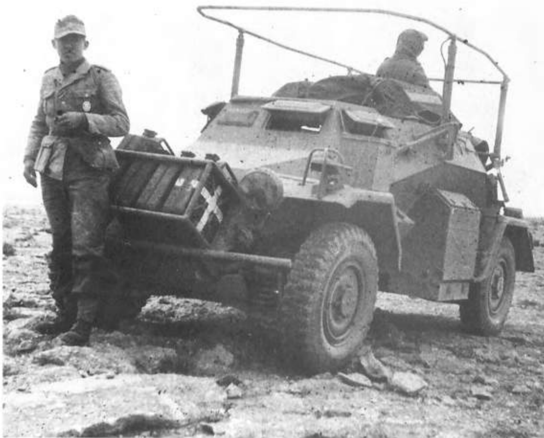
Above: An SdKfz 221 mit 2.8cm gun of 1942. Early scout cars had to be accompanied by an armoured car to provide firepower. However, from 1942 some 220 were fitted with a 2.8cm sPzB41 gun, which had a tapered bore (2.8cm at the breech to 2cm at the muzzle) to increase muzzle velocity. (TM)
