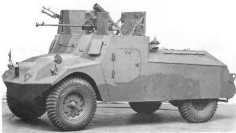
Below: Morris MkII light reconnaissance car, a 4x2 vehicle weighing 3.7 tons with a crew of three and a top speed of 50mph. Armament was a Bren LMG and a Boys anti-tank rifle. (TM)
