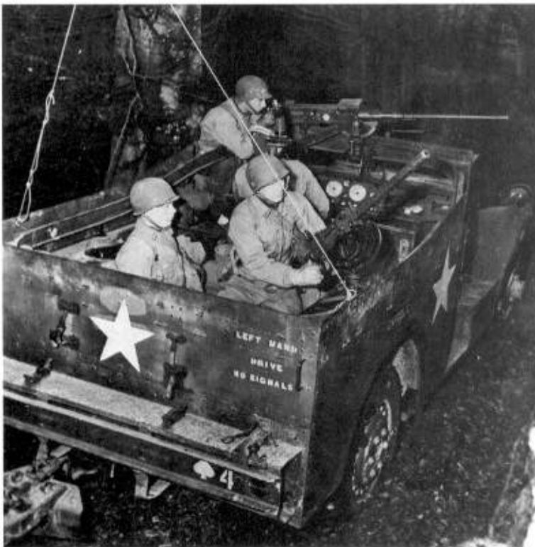
Below: M3A1 scout car fitted with the standard .50in Browning heavy MG at the front and a .30in at the rear, both on pintle mountings. (TM)
