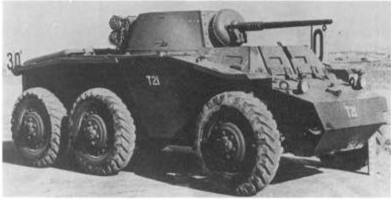
Above and left: Front and rear views of the Studebaker-built T21 6x4 armored car of 1942. It was also designated as the T43 GMC. (TM)
